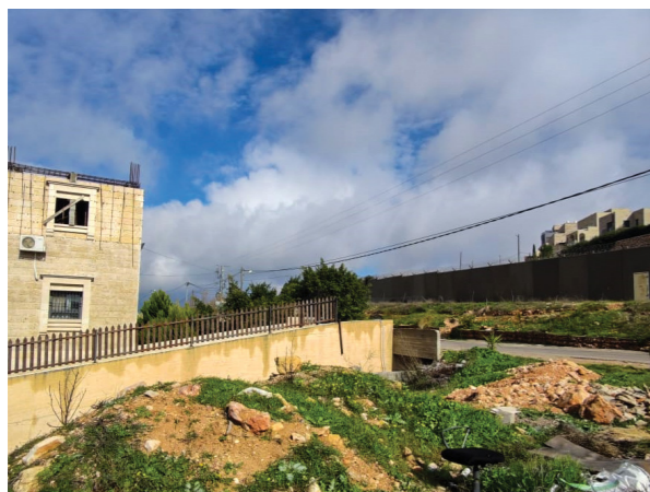
On the right side of the picture is Al Walaja clinic, with the Israeli wall and the Har Gilo illegal Israeli settlement on the other side of the road, equipped with cameras facing the health center. The Israeli military roadblock is just a few meters away. (Médecins du Monde Switzerland, 2024)
